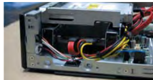
All cables secured with cable ties
